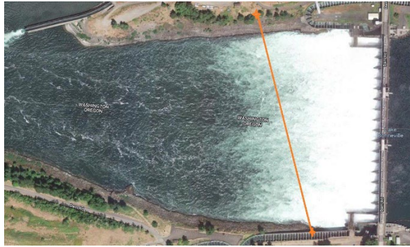
Photo 1. BON broken avian wire location.
